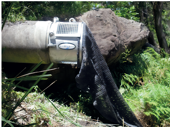
Figure 2: Net over drainage pipe
