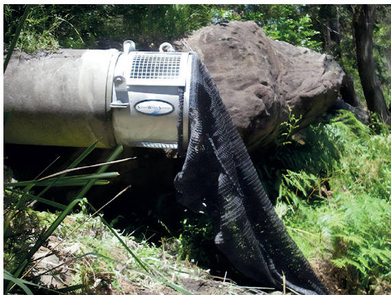
Figure 2: Net over drainage pipe
