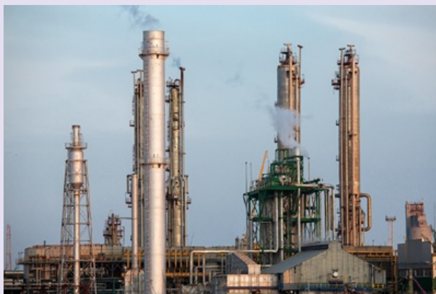
Figure 8.1: Ammonia plant in Western Australia.
