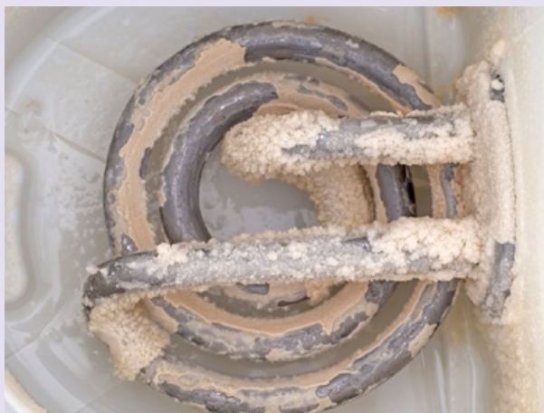
Figure 21.1: In a hard water area, enough limescale is formed in water pipes, kettles and boilers in your house to fill a small bucket!
