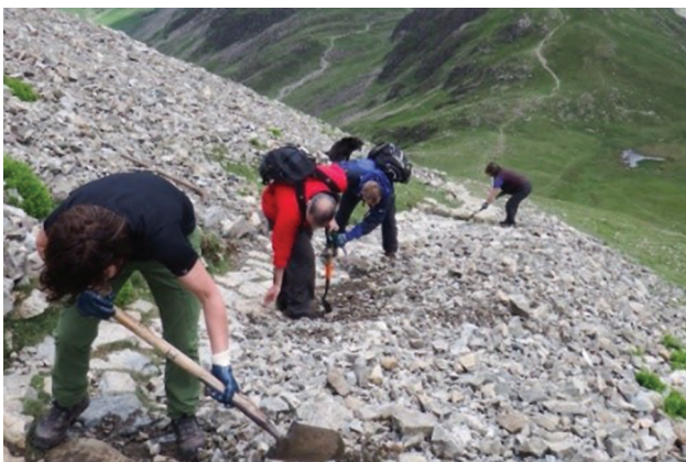
Repairing paths in the Lake District
