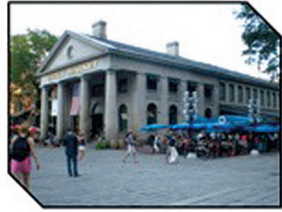
Conservation of built heritage. Re-use derelict buildings.
